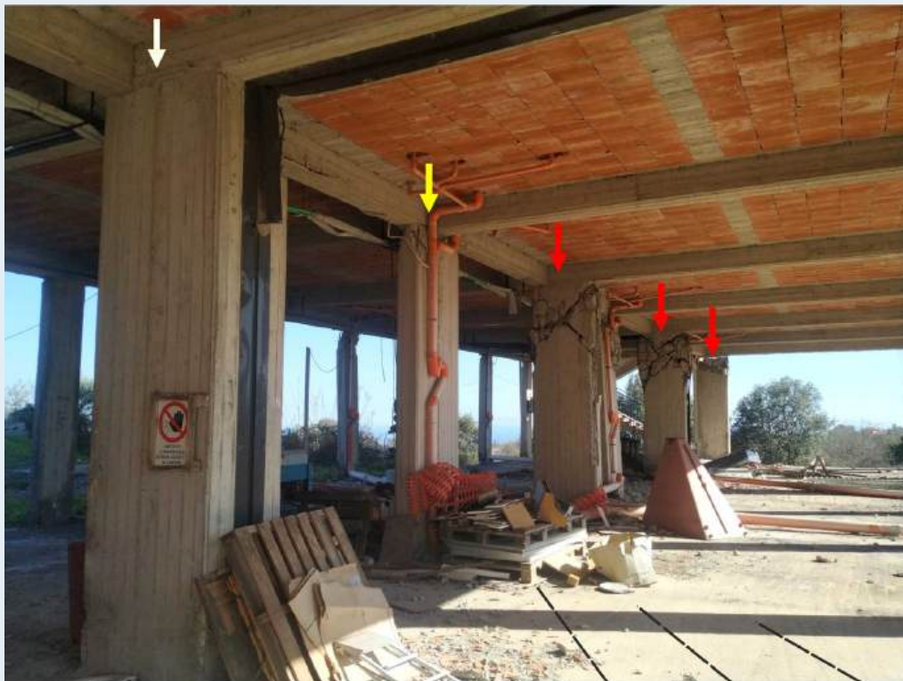
Figure 6. The building has been displaced by the action of the ACF. The damage is selective in nature, with the reinforced concrete columns failing at the junctions with the first floor (red arrows) in the section of the building constructed above the fault (black dotted lines, bottom). As one moves away from the fault line to the left, the columns exhibit less damage (yellow arrow) or no damage at all (white arrow).
